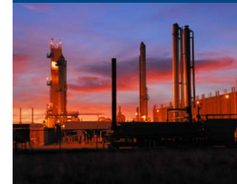
Integrated Energy Systems
