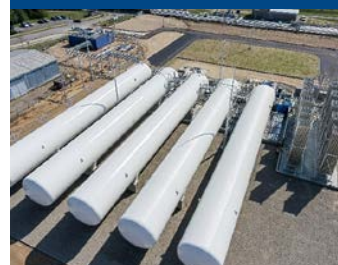
Cryogenic Storage & Regasification Systems
