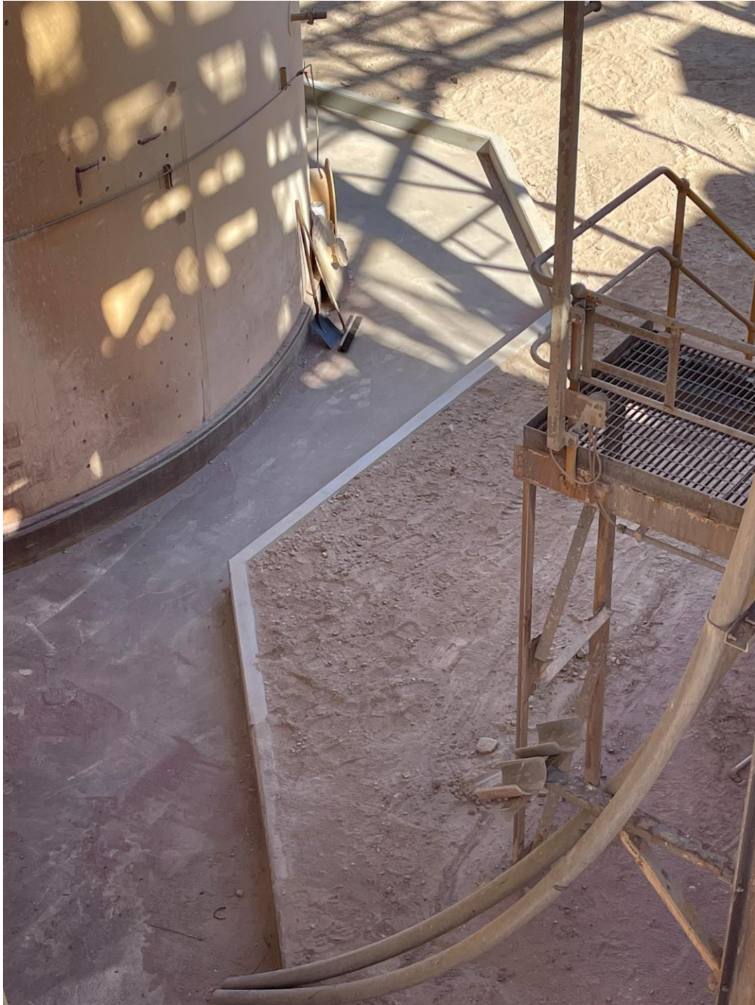
(Figure 3: Completed concrete repairs to the tank bund walls - view facing north east.)
