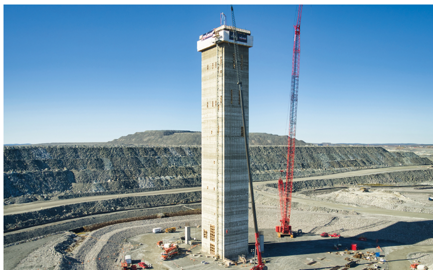
Figure 1: Production shaft construction at Odyssey - Click here for more details
