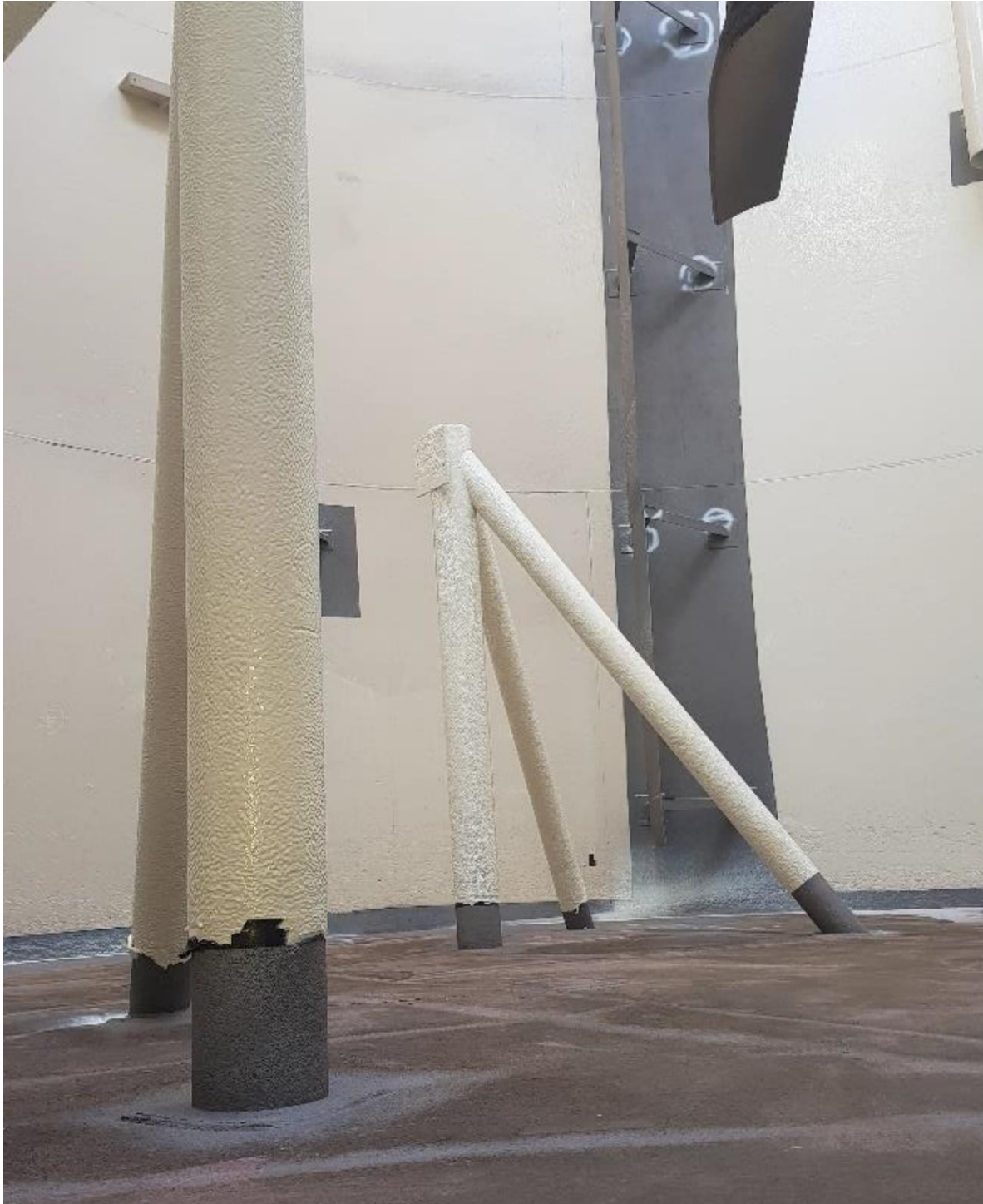
(Figure 4: Tank internal painting partially completed.)
