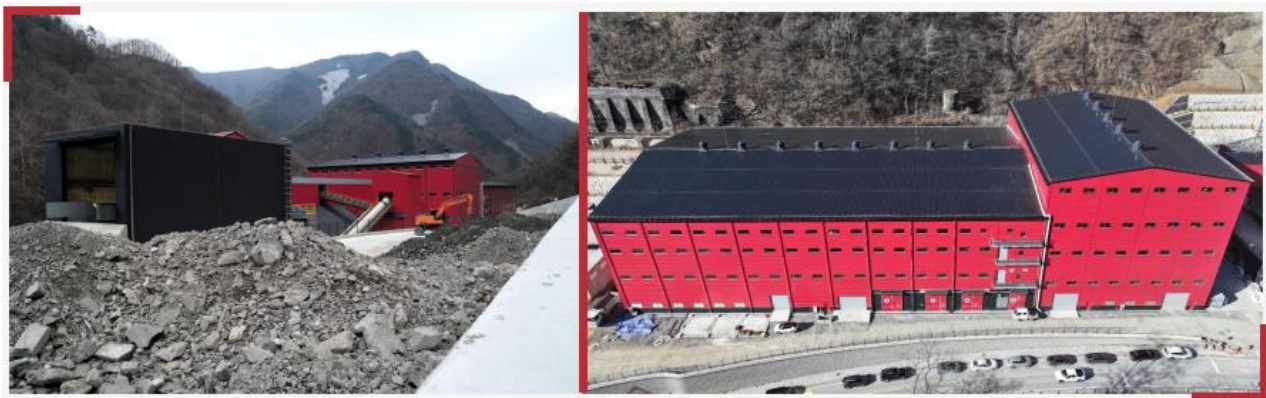
Exhibit 5: Sangdong Tungsten Mine Construction Impression as of January 2026. Source: Investor Presentation
