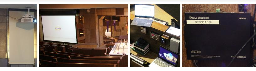
controllable device. The KD-IP922 is a completely flexible and expandable system, where a single encoder was added for each of their video sources and a single decoder for each display and projector. Not only was Key Digital's AV over IP system perfect for updating the AV system at Shrine of the Little Flower, it is also the perfect fit for the church's requirements.
