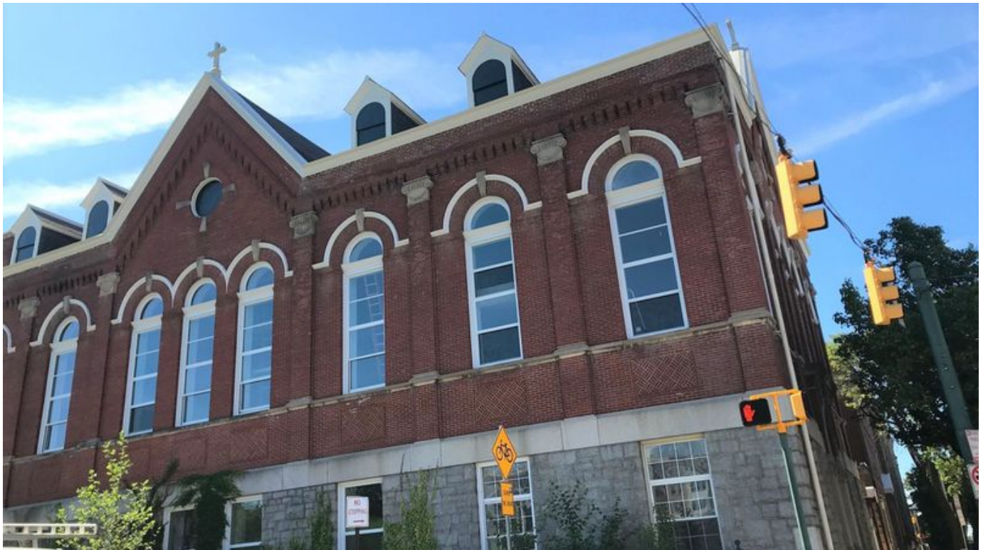
The parish hall, girls school and rectory at old St. Michael's are being converted into apartments while the church becomes a brewery. (Baltimore Sun)
