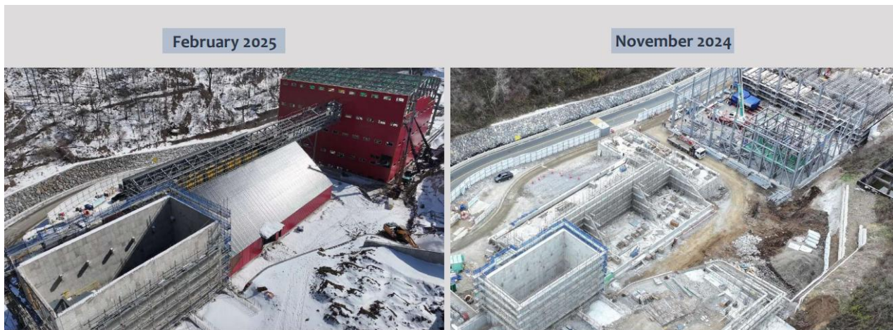
Exhibit 5: Sangdong Tungsten Mine Construction Impression as of February 2025. Source: Investor Presentation
