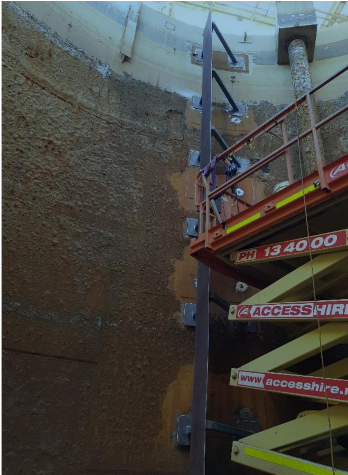
(Figure 3: Replacement baffle installed in tank prior to completion of water blasting and painting. Note the extensive corrosion on the tank wall)
