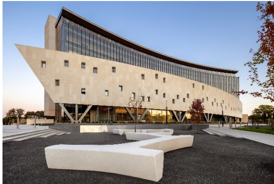
Johnson County Courthouse. Photo: © Bill Timmerman
