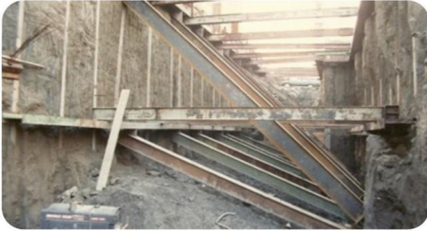
Figure 5: Internally braced excavation adjacent to a building, Toronto.
