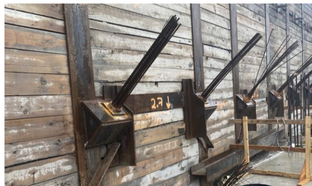
Figure 4: Steel tieback cables protruding from and attached to a retaining wall; view from within the excavation.
