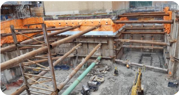
Figure 7: Site braced with steel props due to lack of permission to install tiebacks, Toronto.
