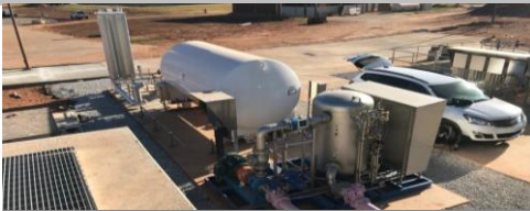
Liquid oxygen for wastewater treatment (Wichita Falls, TX)
