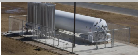
Liquid oxygen system for ozone generation (Duchense, UT)
