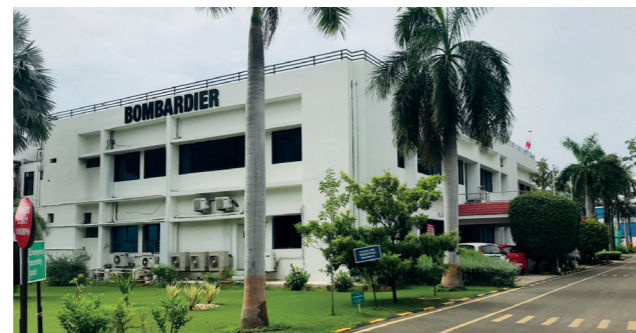
2 Bombardier's Maneja site in Vadodara will provide propulsion control and electrical systems
