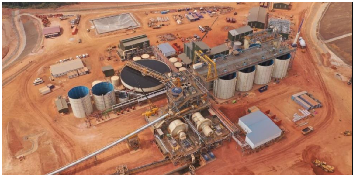
Picture 1: Process Plant
