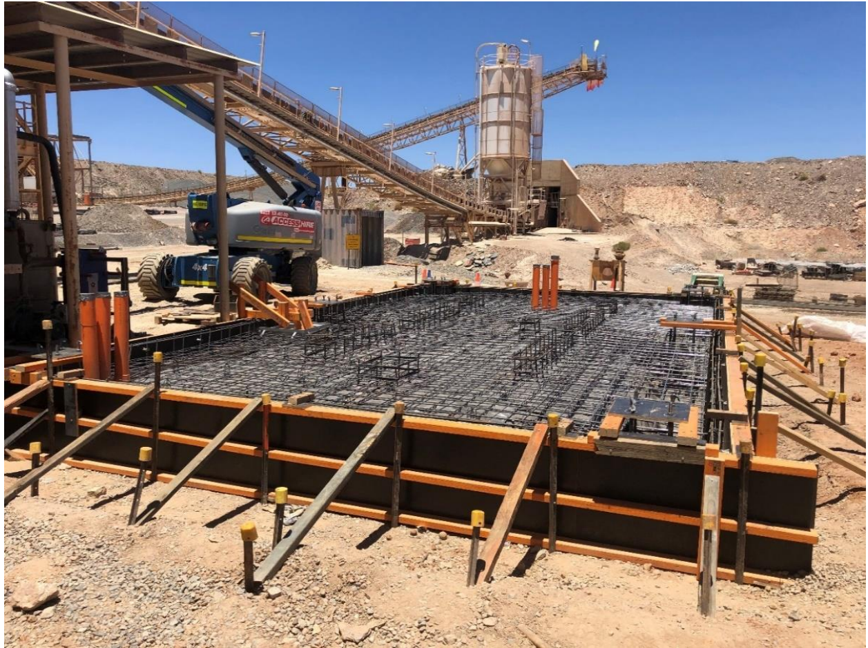
(Figure 4: Foundation for the new Acacia reactor unit being prepared for first concrete pour – view facing south.)
