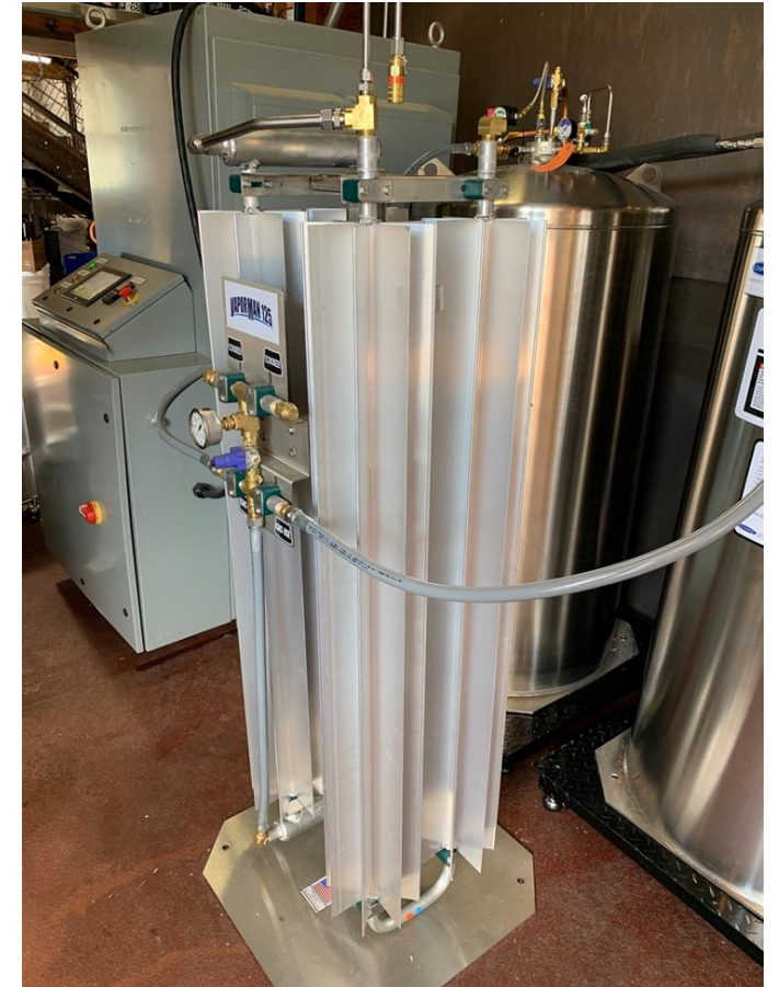
2 1,000 lb Tanks and Vaporman to Right of Installation
