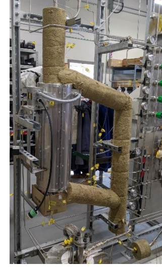
FLiBe Corrosion Loop
