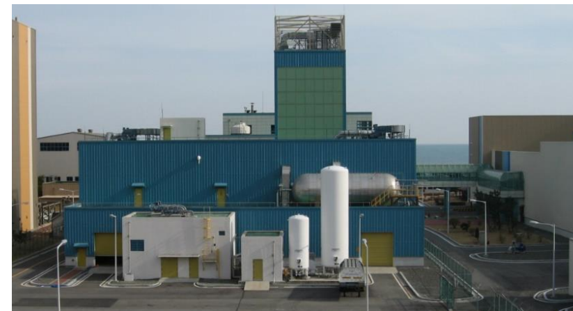
Industrial Scale Water Detritiation Facility
