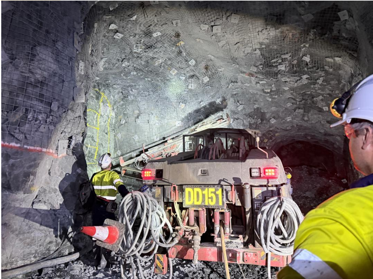
Figure 2: Underground development activities at CMA
