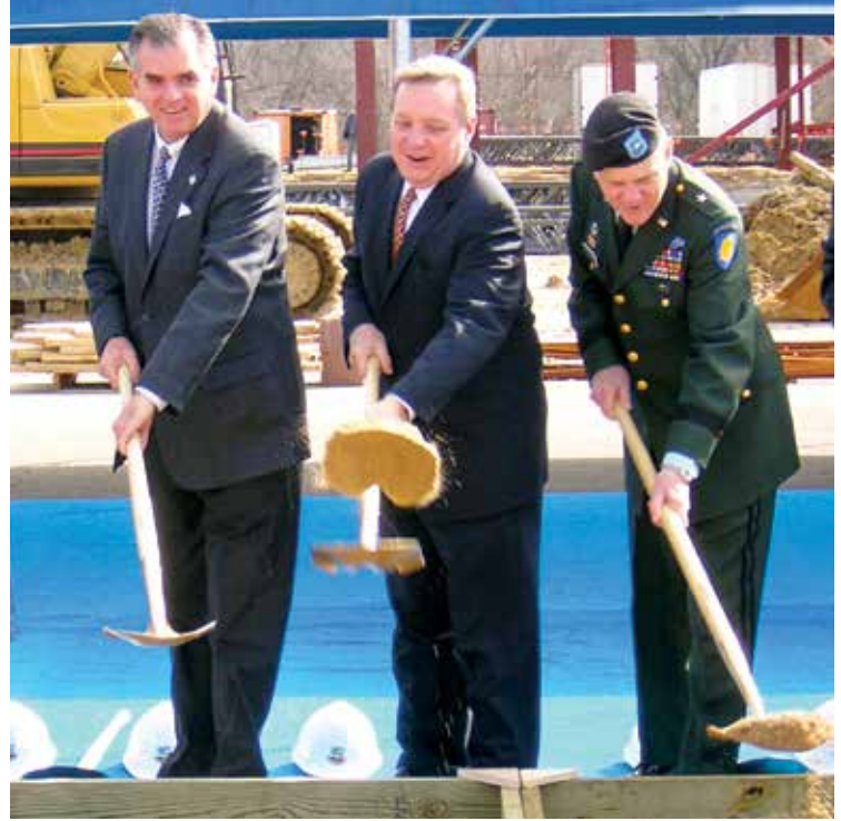
Then-U.S. Rep. Ray LaHood and Sen. Dick Durbin break ground on a new National Guard facility in the 18th Congressional District.
