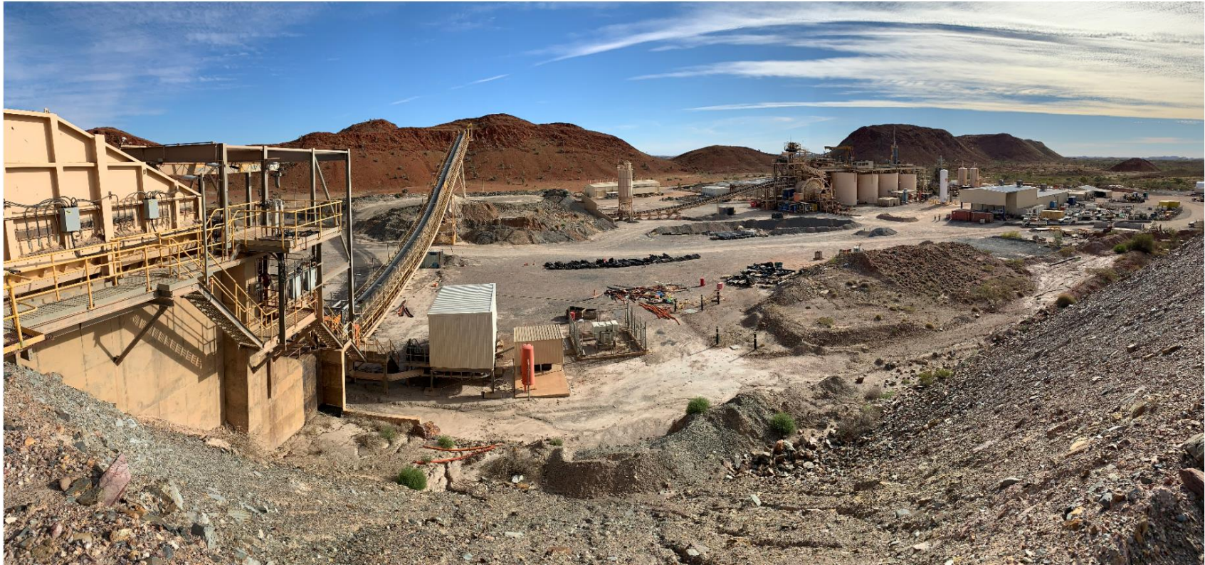
(Figure 3: Nullagine processing facility.)
