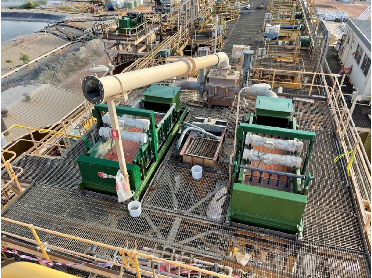
(Figure 3: Fully refurbished and re-installed trash screens on the Golden Eagle Mill.)
